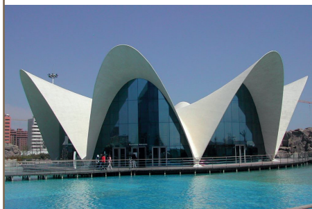
Steel fiber reinforced concrete thin shell structure Oceanographic Park Restaurant. City of Arts and Sciences, Valencia (2002) Based on blueprint of Felix Candela, by: A. Domingo, C. Lázaro, P. Serna
